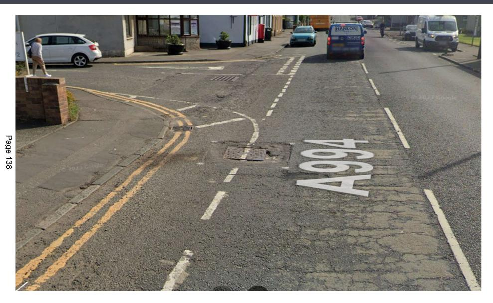
Figure 7: Road markings at junction to assist with visibility - Cairneyhill
